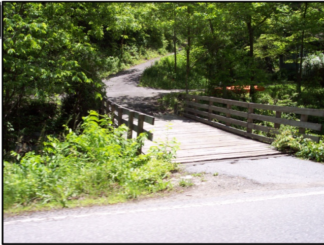
Bridge serving as a driveway on Hayes Run Road
