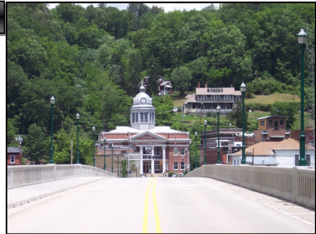
Bridge crossing the river into Downtown
