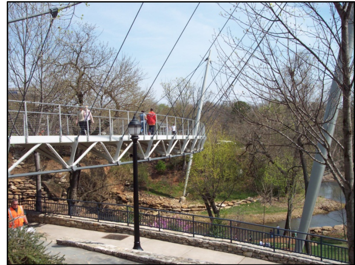
Reedy River downtown park pedestrian bridge, Greenville, SC
